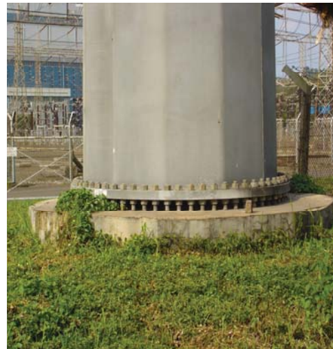
Gambar 4. 16 Pondasi steel pole 500 kV dead end Suralaya
