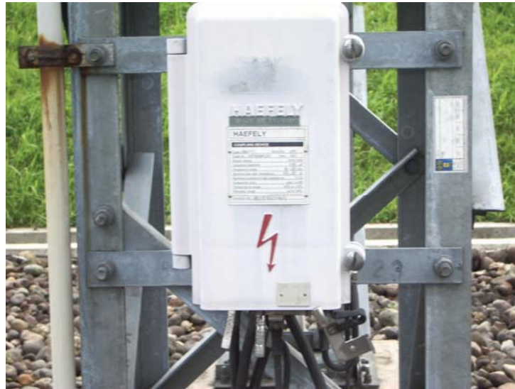
Gambar 5.39. Coupling Device
