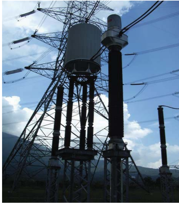
Gambar 5.41. Wave Trap 500 kV
