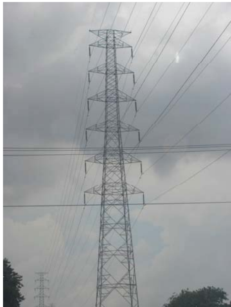
Gambar 4.8 Tower 4 sirkit tipe suspensi tipe tension
