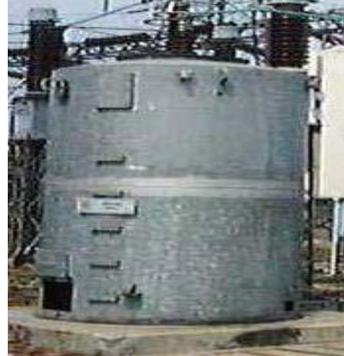
Gambar 5.8. Resistor Jenis Cairan ( liquid resistor )
