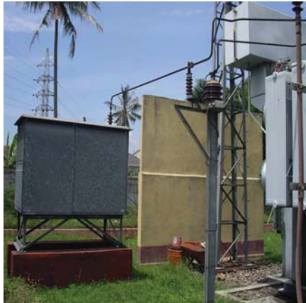
Gambar 5.6 Resistor Jenis Logam ( metallic resistor )
