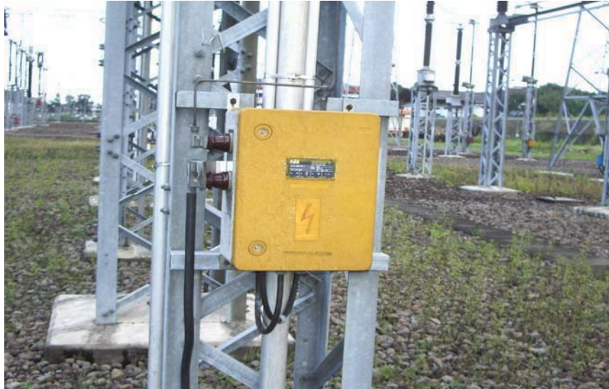
Gambar 5.46. Line Matching Unit
