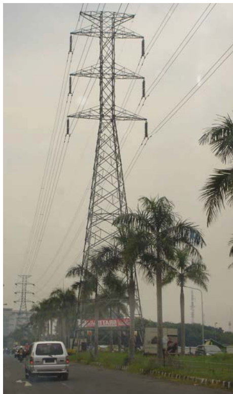
Gambar 4.10 Tower 2 sirkit tipe suspensi
