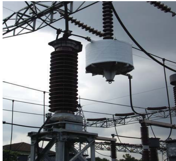
Gambar 5.40. Wave Trap 150 kV
