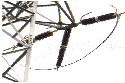
Gambar 4.32 Tension clamp
