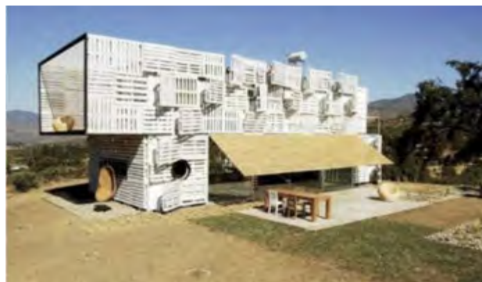
Gambar : Manifesto Huose, Green Home Made of Wood Pallets and Shipping Containers L Recyled Home
