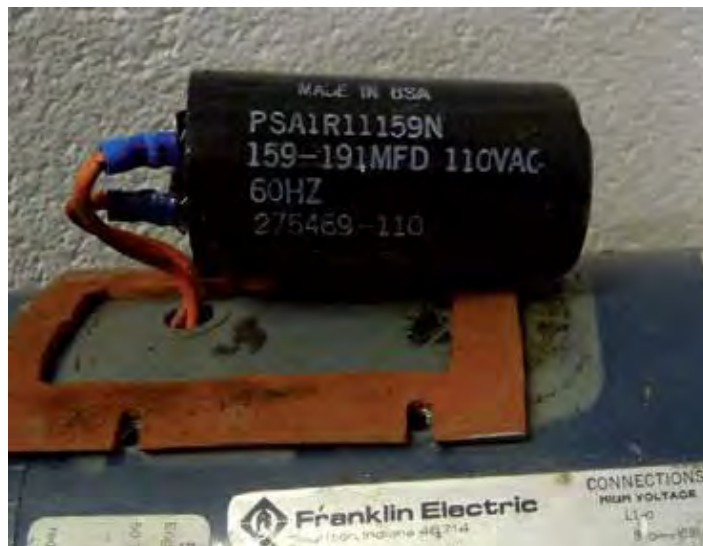
Gambar 5.3 Tipikal Starting Capacitor (159-191 mfd)
