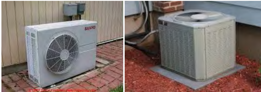
Gambar 6.7 Pemasangan Unit Outdoor
